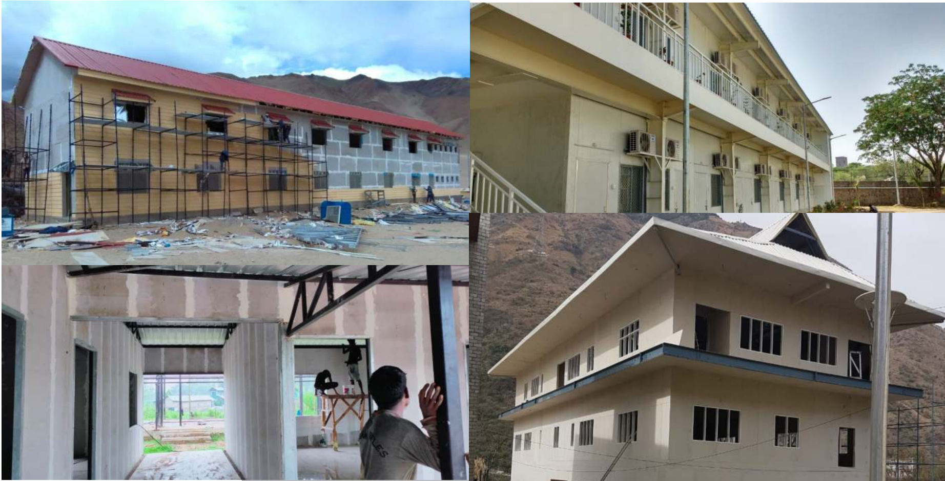
Army Residential Quarter & Offices
